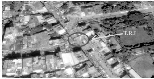
Figure 1.1(a): Trunk road intersection point (Source: Google Map)
