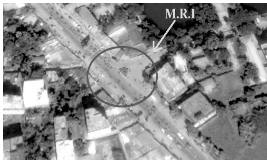
Figure 1.2(a): Mizan road intersection (Source: Google Map)
