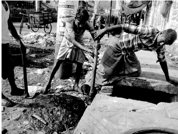
Figure 6: Sewerage maintenance in Feni town.
